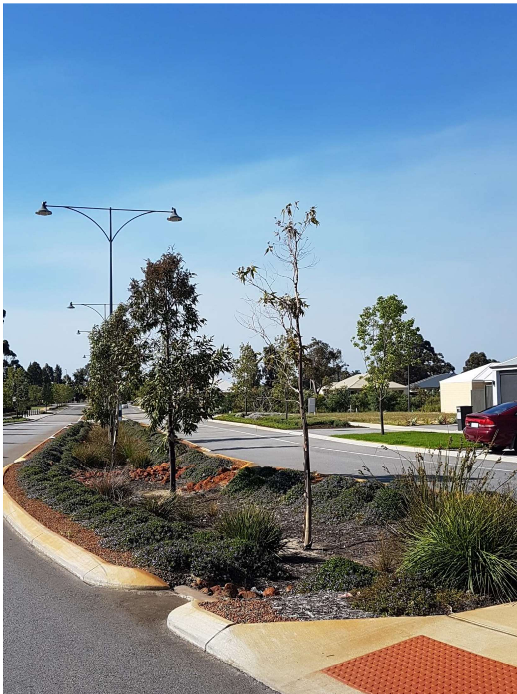
Figure 14: Example median swale arrangement
