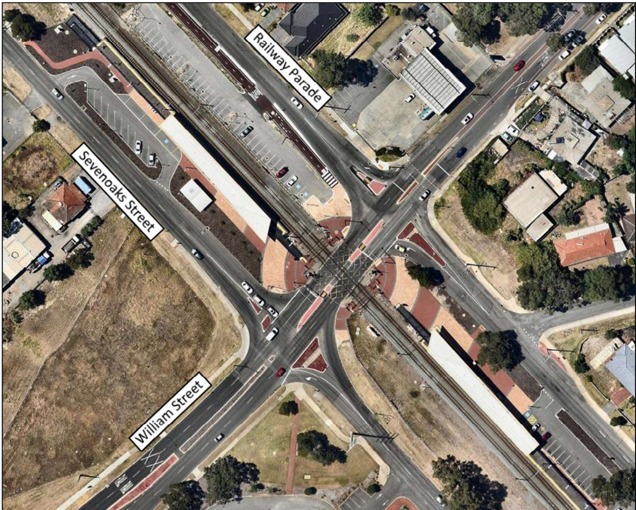
Figure 3-3 Level Crossing at William Street / Sevenoaks Street / Railway Parade
