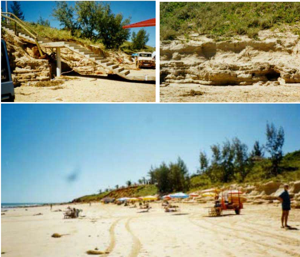
Figure 6.7: Cable Beach eroded base of dune post Tropical Cyclone Rosita 2000 (JCU 2000).
