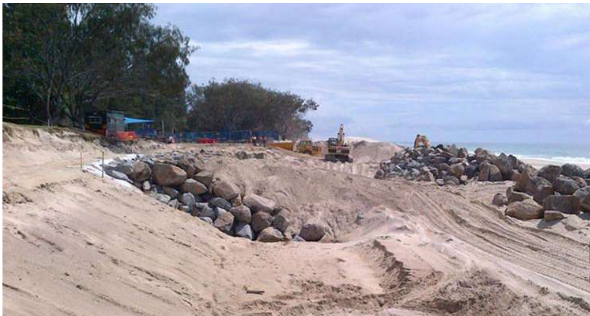
Figure 6.5: Buried Seawall under construction (GCCC 2016)
