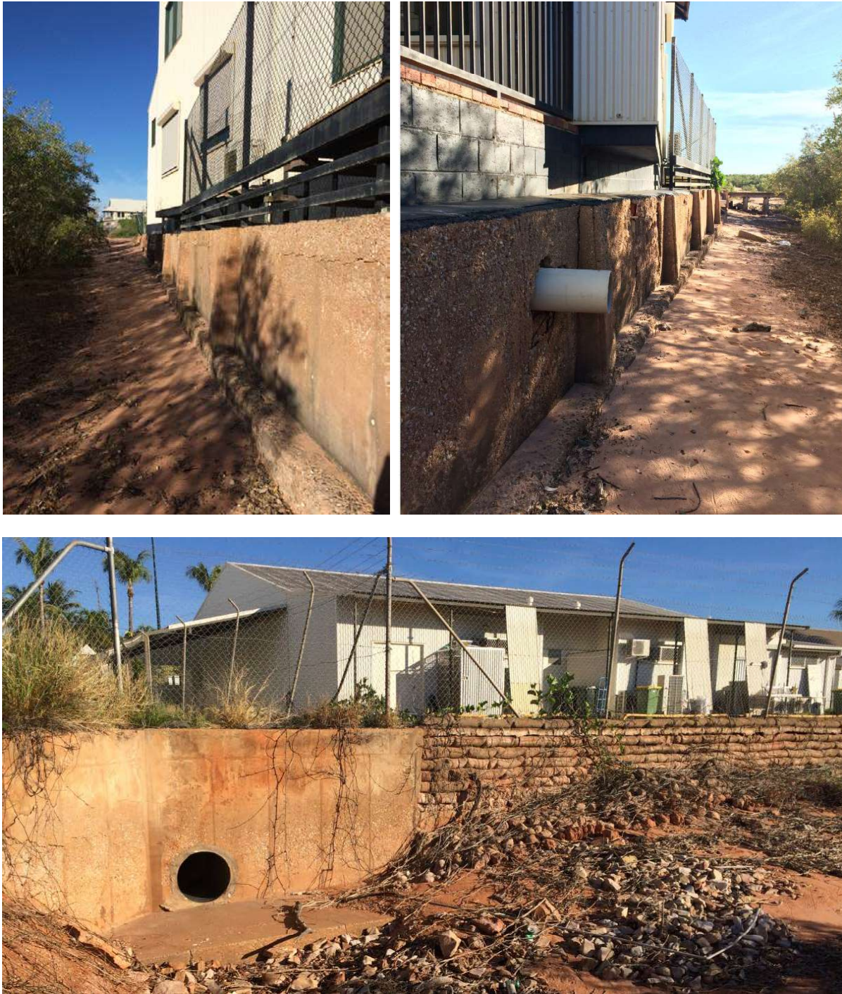
Figure 3.7: Seawall / revetment in the Dampier Terrace shoreline south of Streeters Jetty
