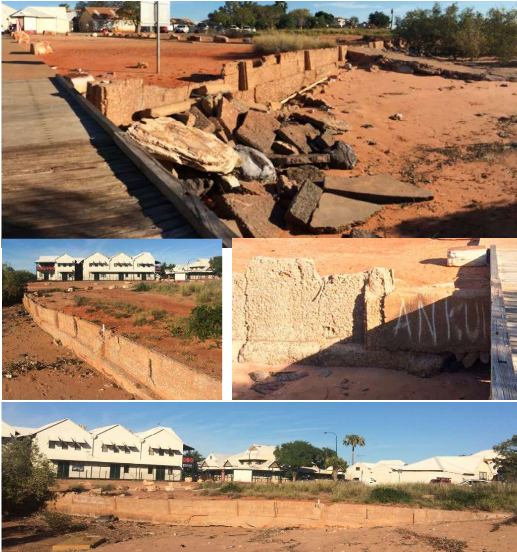
Figure 3.6: Seawall / revetment in the Dampier Terrace shoreline north of Streeters Jetty
