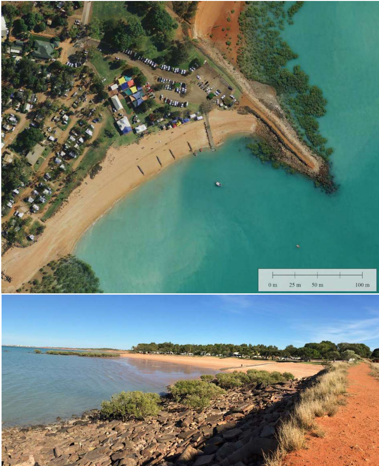
Figure 3.5: Old Broome Jetty Groyne Structure, Town Beach
