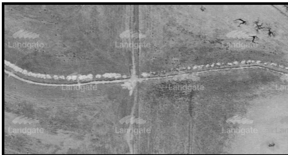
Plate 2: St Leonards Creek Excavation in 1965
