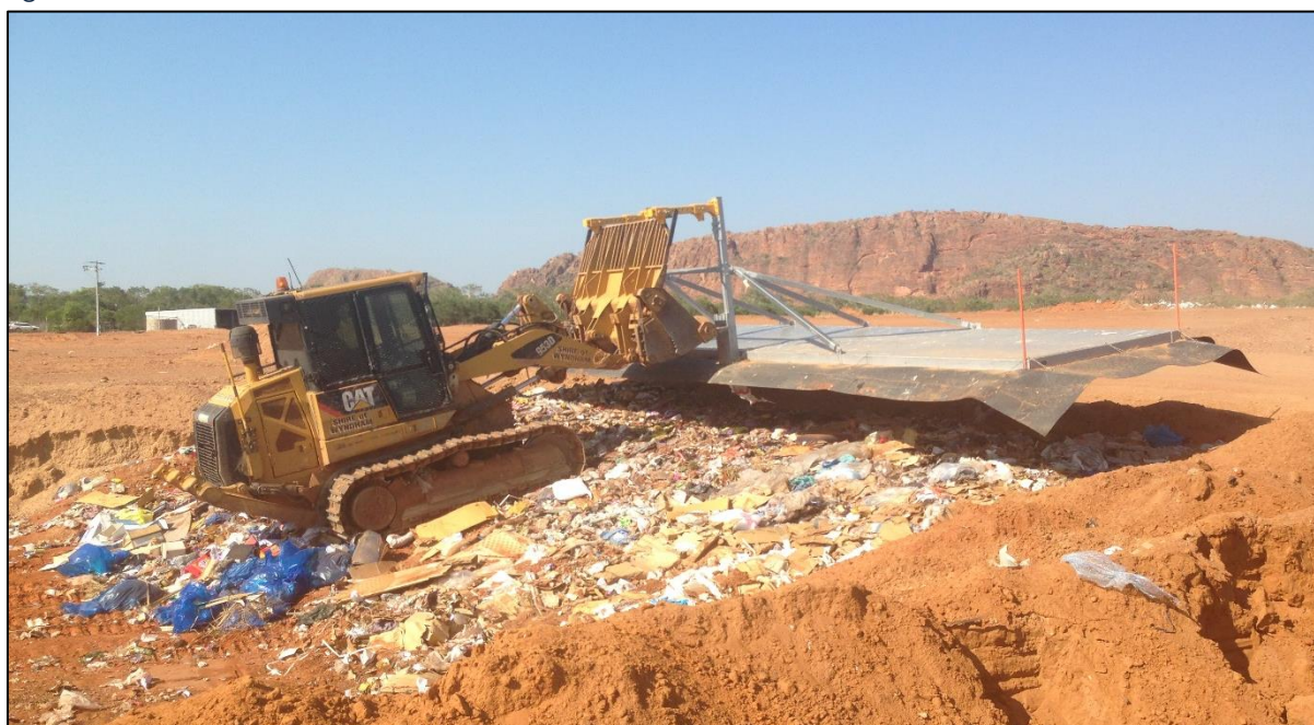
Figure 5.1 - Tracked loader and landfill lid
