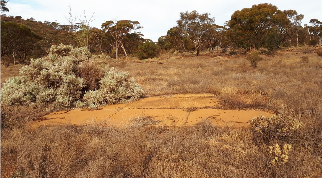
Photograph 4.2: A concrete slab, formerly associated with a house, in the area proposed for expansion of the warehouse and yard.
