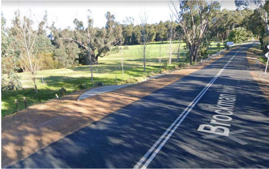
Existing pathway connecting Cockatoo Valley subdivision south of Nannup town site Brockman Highway. Proposed pathway to join up with existing pathway.
