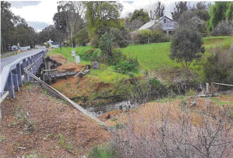
Photo 4: Services at Abutment 1 LHS on Bridge 0256A (as viewed from Abutment 2)
