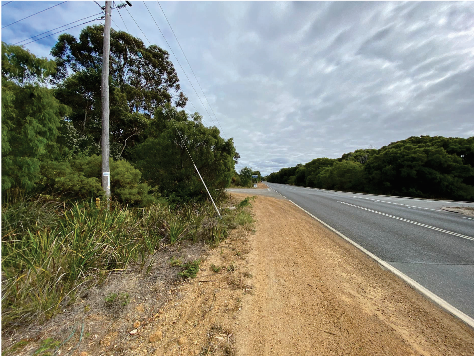
Looking NW towards the crossover (including the 1 st Power pole).
