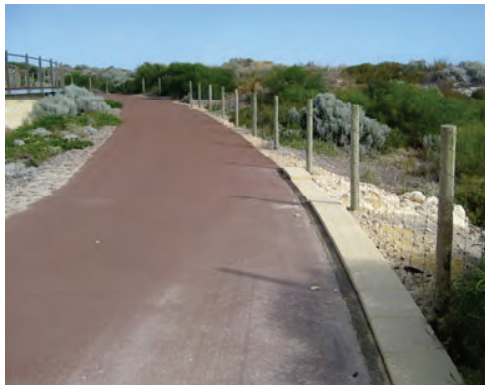
Figure 9: Stage 1 Dual Use Path – 3m wide red asphalt. Note limestone kerb to control minor drainage and galvanized wire and treated pine fencing to all sides(unless otherwise contained).
