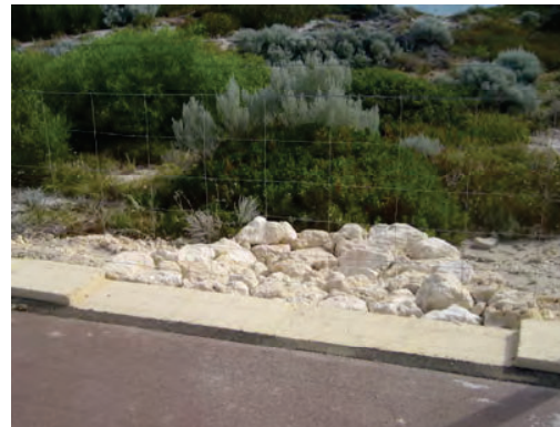
Figure 9: Stage 1 Dual Use Path – 3m wide red asphalt. Note limestone kerb to control minor drainage and galvanized wire and treated pine fencing to all sides(unless otherwise contained).
