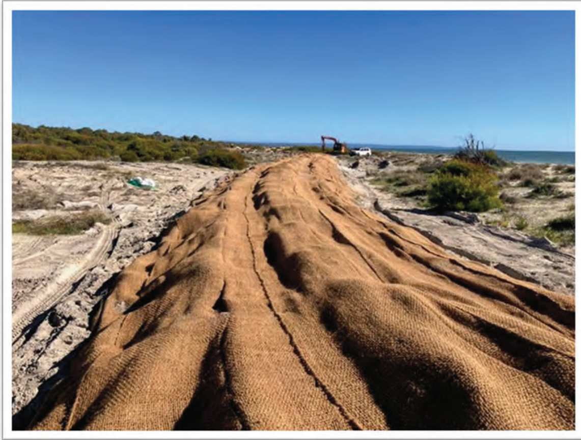
Plate 3. Coir matting to prevent wind erosion.
