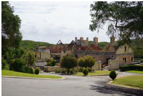
Plate 2: Cleared and parkland cleared areas of the site including Wallcliffe House.
