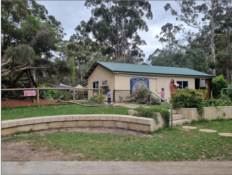
Fig.3 – Photo of the branch that failed and fell into the target area of tree #G01D on 26/11/2024. (Photo provided by Kwoorabup Nature School by email on 17/12/2024).
