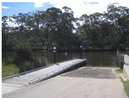
R: Denmark floating jetty Launch
