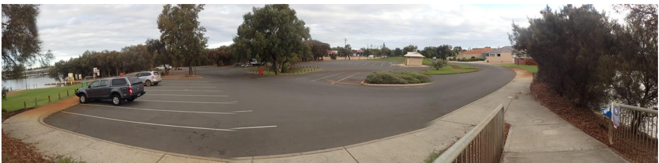
Mix of 'drive through' and 'nose in' trailer parking at Riviera Way boat ramp Bunbury
