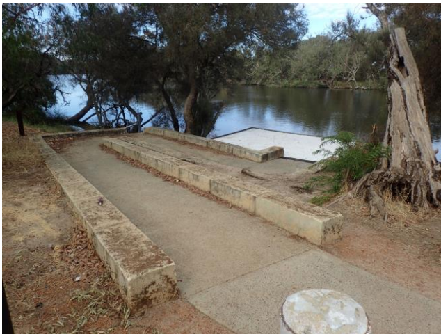
L: Wheelchair ramp to a fishing platform, and
