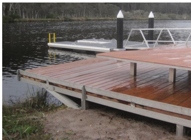
R: Low cantilevered deck at Nornalup
