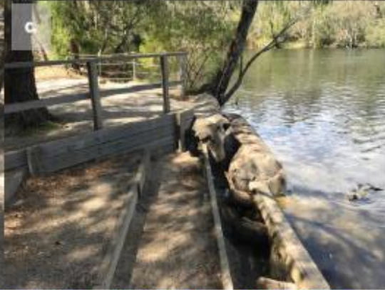
River Access 3 including a) compacted gravel stairs with timber supports, timber retaining walls and handrails, b) failed lower stair and undercutting of timber retaining wall on upstream side, and c) timber logs for bank protection downstream.
