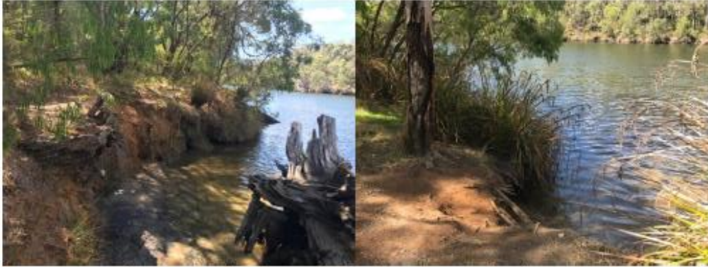
Downstream river banks showing variable elevation, embankment undercutting and informal access.
