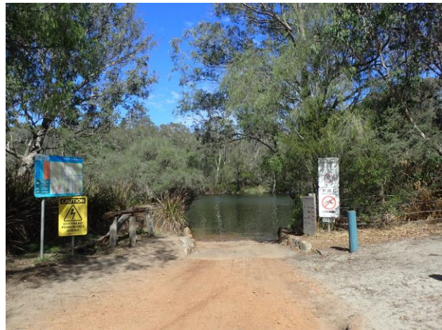
L: problems getting on and off boats and bank erosion R: Narrow ramp, hard for backing, worn edges
