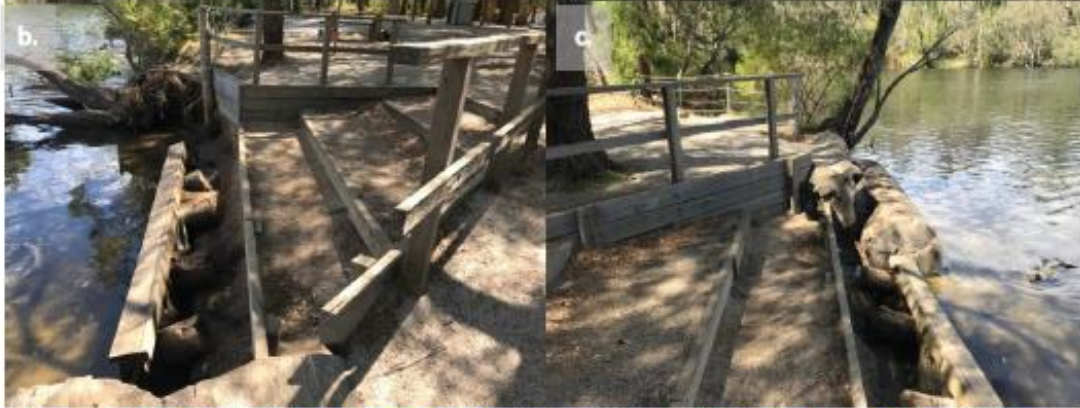
River Access 3 including a) compacted gravel stairs with timber supports, timber retaining walls and handrails, b) failed lower stair and undercutting of timber retaining wall on upstream side, and c) timber logs for bank protection downstream.
