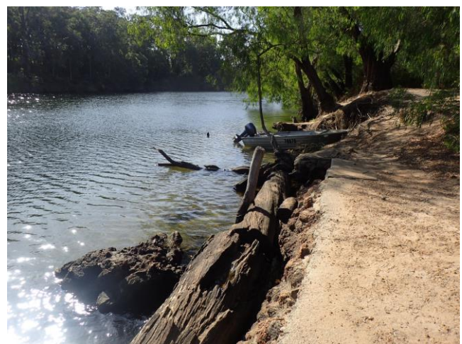
L: Undercut toe of access structure is hazardous for pedestrians R: Undercut cemented rock wall with void
