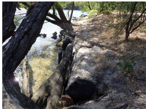
L: Log with no scouring at toe or behind log, gentle bank and fence R: Log with second log for toe scouring
