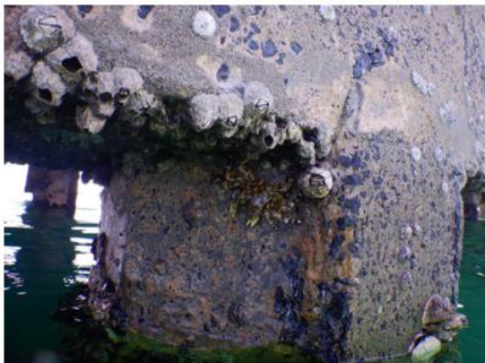
Figure 4 Typical condition of concrete piles
