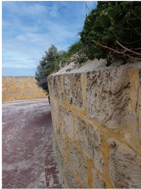
Plate 19: Example 1 of top end of limestone wall beginning to bend from the weight of the sand dunes.
