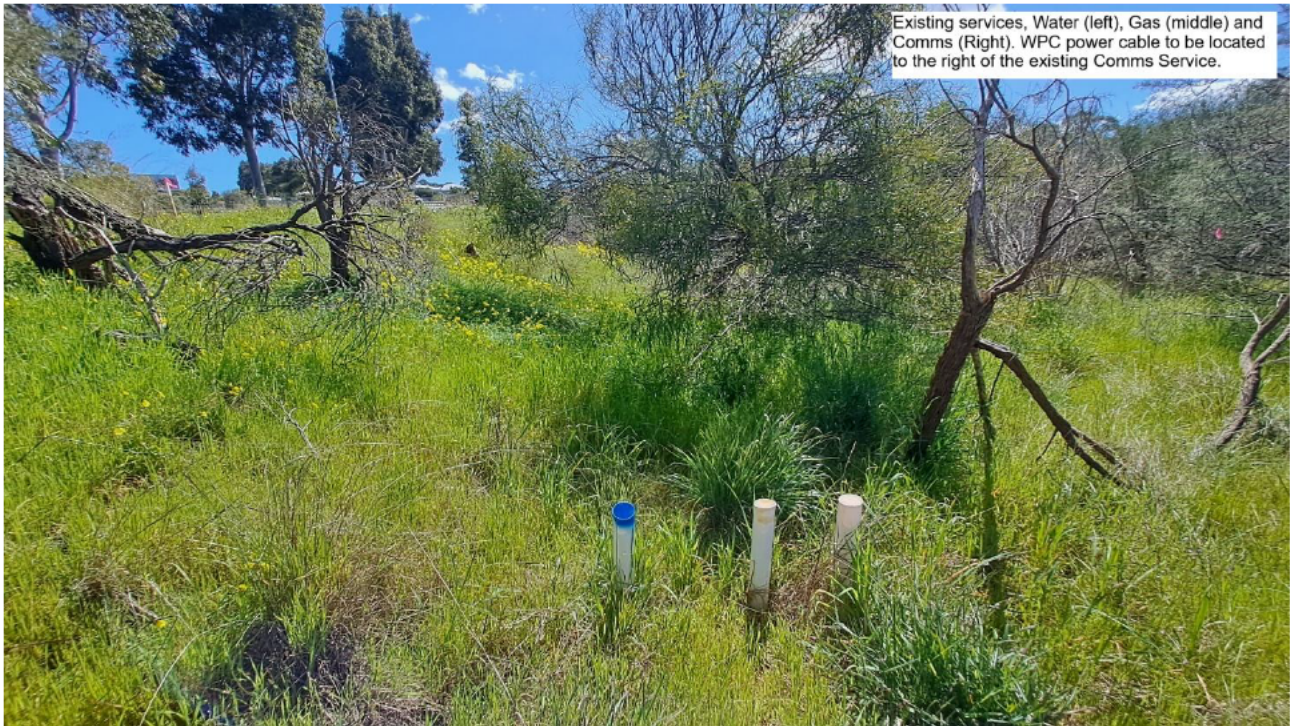
Plate 1: View looking north, close to points C-F, showing existing service locations, water, gas and comms.
