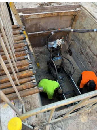
Figure 6: Example of works showing the drill rig in the pit.
