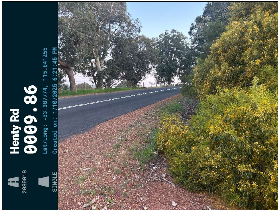
Finding 2.7 – The access at this location has a restricted sight distance due to the vegetation. The vegetation should be trimmed to provide suitable sight distance.
