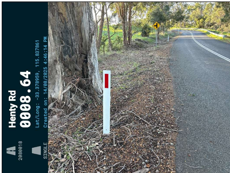
Finding 2.2 – The large tree stump is close to the traffic lane and should be removed.
