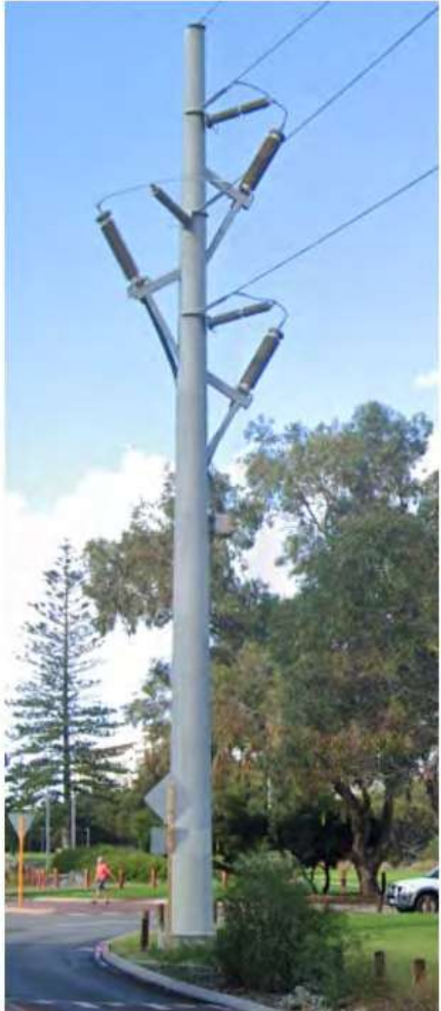
Figure 8: Underground cable to overhead line Transition pole
