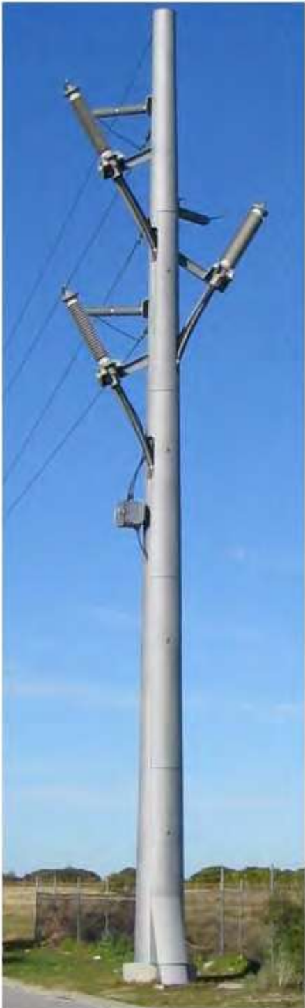
Figure 8: Underground cable to overhead line Transition pole
