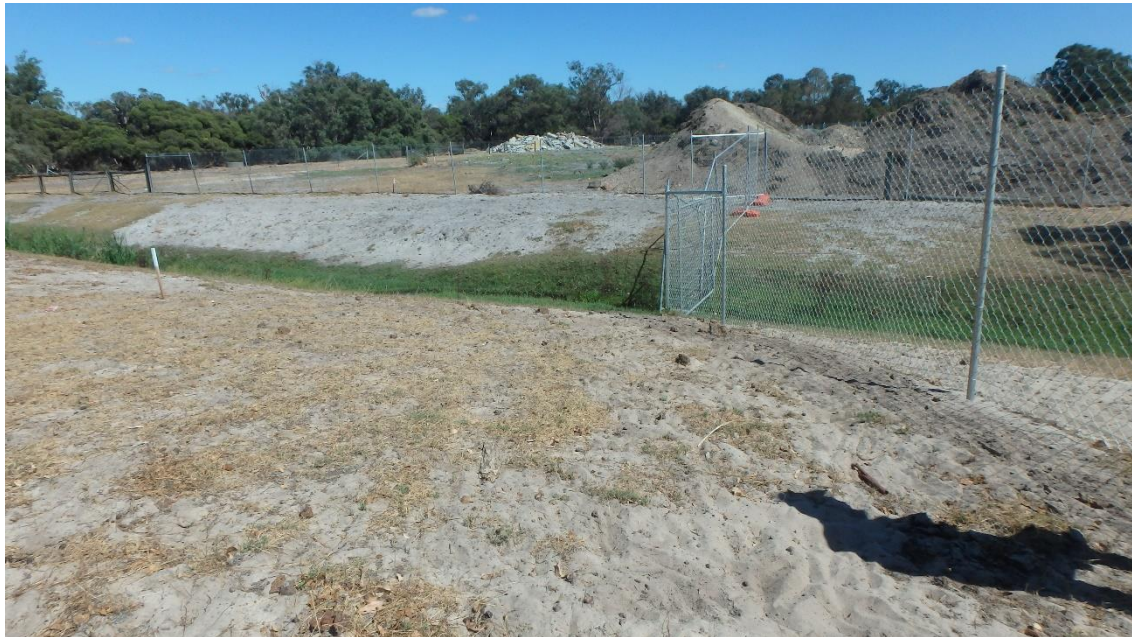
Plate 1: Plant community Cc./Mp./Er.Cleared in a 'completely degraded' condition within the site.
