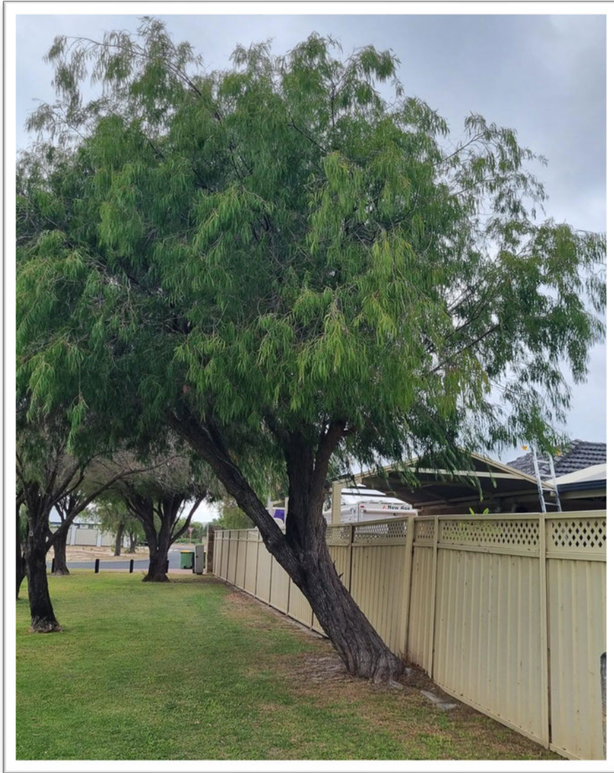
Plate 1. The mature Agonis flexuosa tree subject to clearing due to structural damage of private property.
