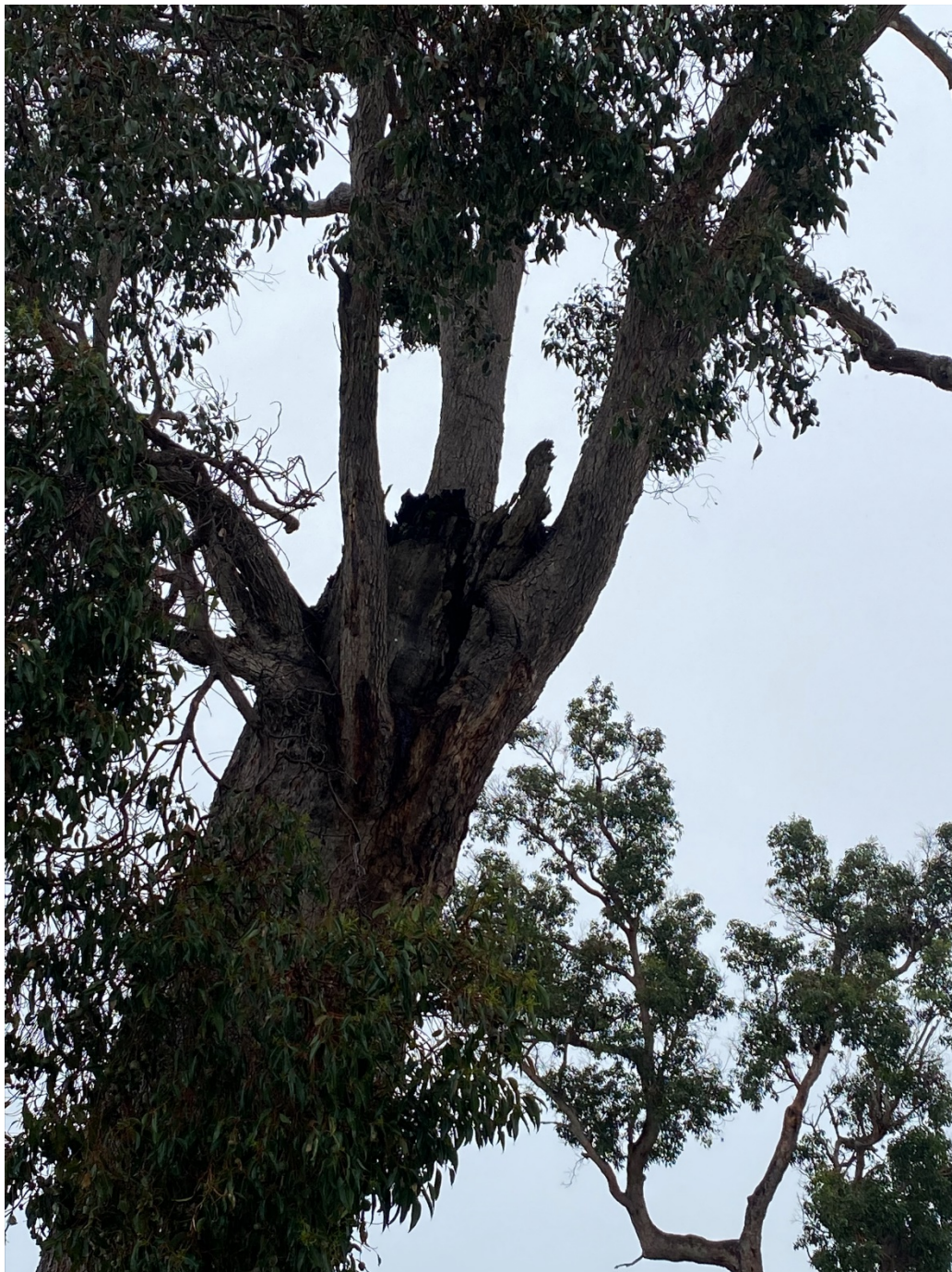
Photo 1: Evidence of major failure to trunk. Weak connections on regrowth also present.
