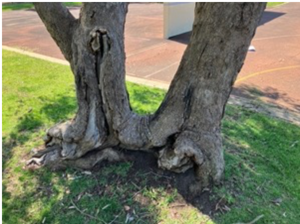
Figure 3: The unusual form of the base of the tree
